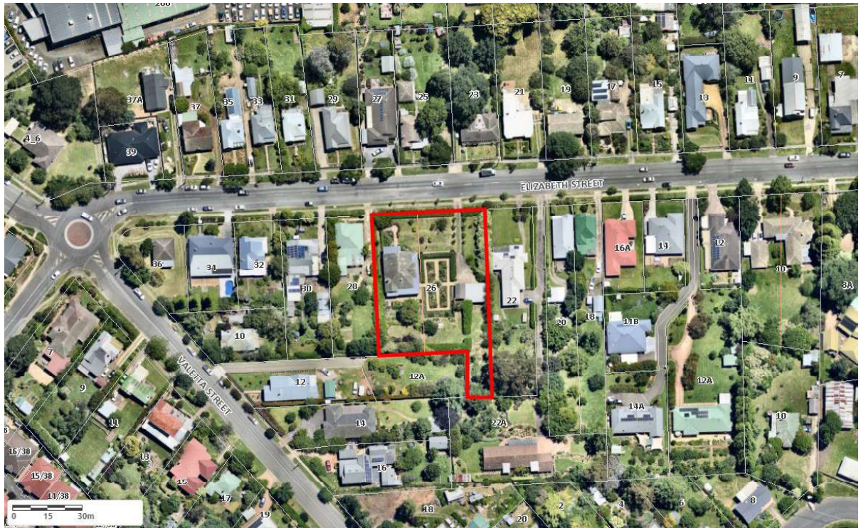
Figure 6: 'Karingal' (outlined) in the context of Elizabeth Street (Source: Nearmap, December 2021).
