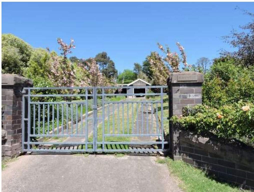
Figure 4: Detail of entry gate with aesthetically significant brick and trachyte fence (Photo by B. Townsing, 2020).
